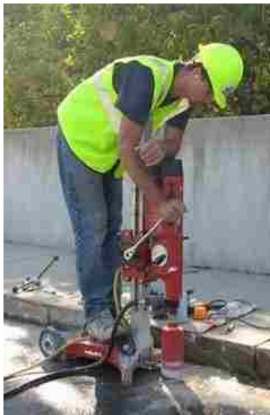
Figure 5.30. Concrete core extraction from Southview Bridge
