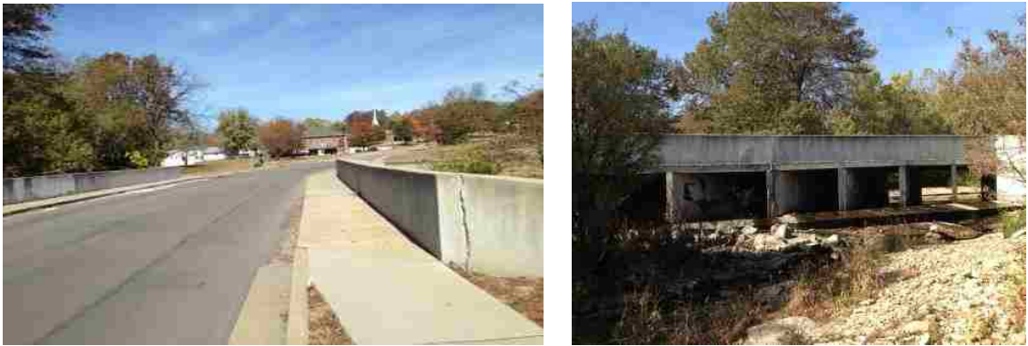
Figure 5.7. View of the new structure
