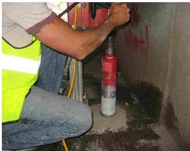
Figure 5.32. Concrete core extraction from Walker Bridge
