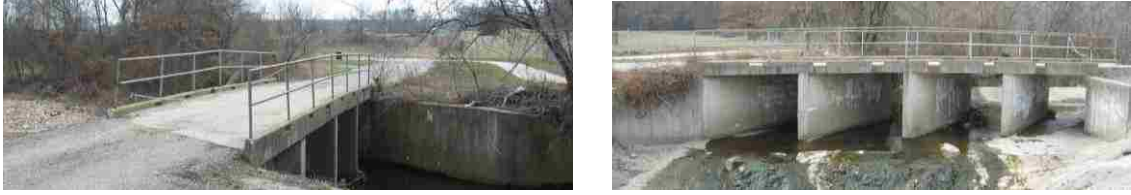
Figure 5.6. View of the existing Southview Bridge [120]
