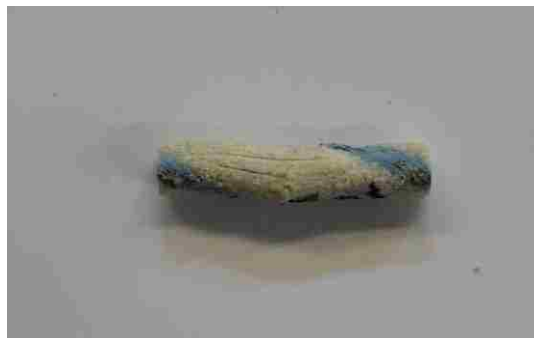
Figure 5.44. Failure #2 GFRP bars from core C-2 B-3 of Walker Bridge
